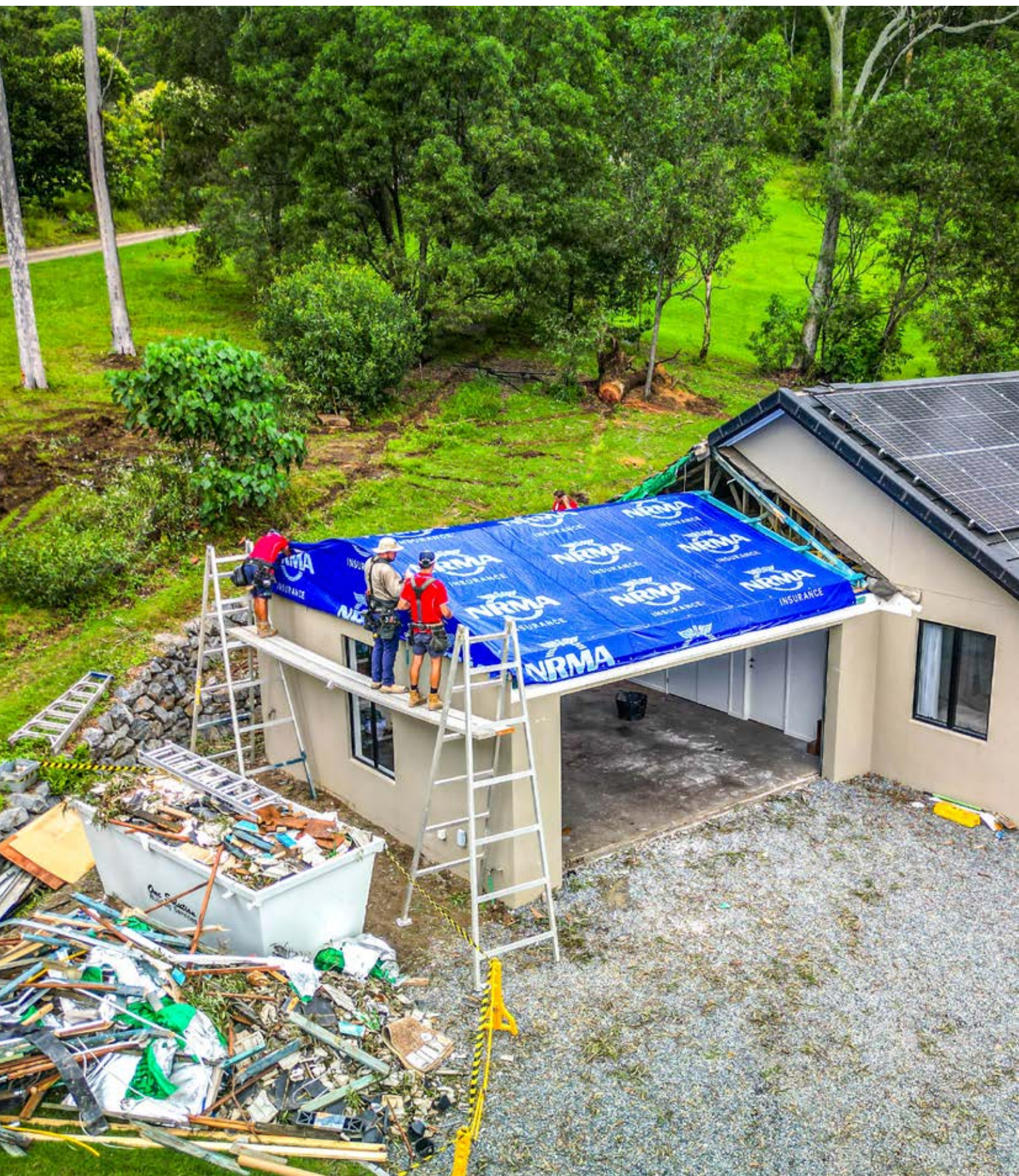
Make Safe roof repairs on NRMA Insurance customers home after Tropical Cyclone Alfred, Gold Coast.
